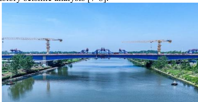
Fig. 1. Beijing-Hangzhou Grand Canal Bridge (Xuzhou Eastern Bypass Expressway)
