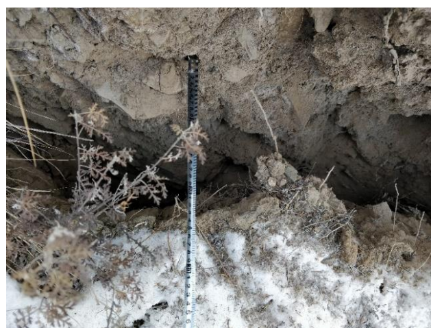
Fig.5 Photographs of the current condition of tension crack IV
